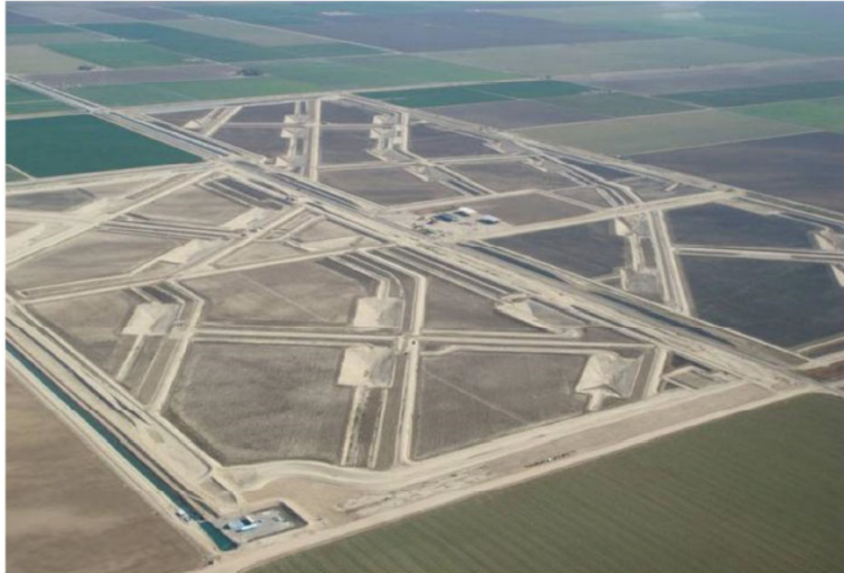
Figure 3.2 Constructed Spreading Ponds for Groundwater Recharge (Semitropic WSD).
